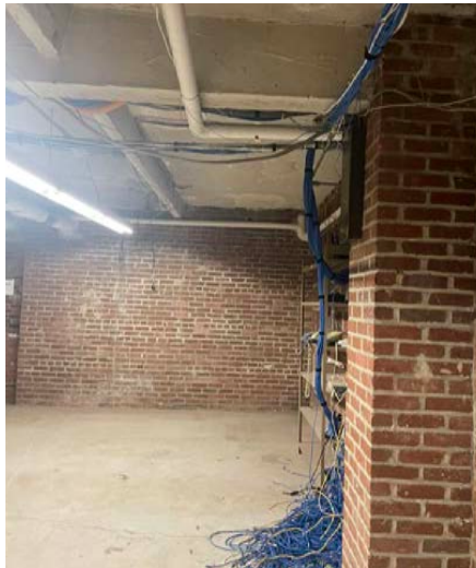
Typical existing condition of lower level
