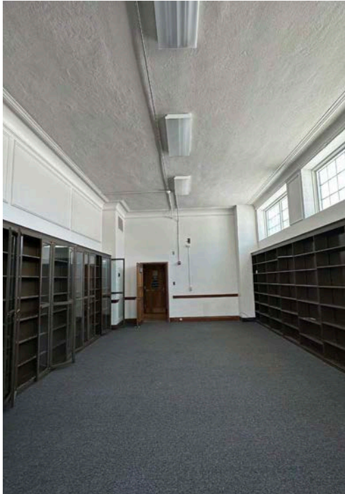
Existing upper floor library space
