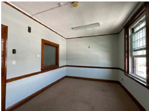
Typical condition of upper floors
