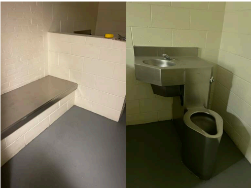
Typical holding cell restrooms
