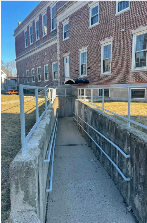
Existing ramp to be modified for new main entry ramp
