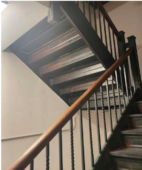
Existing stair to be removed
