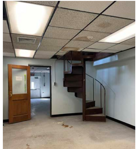
Typical existing condition of lower level
